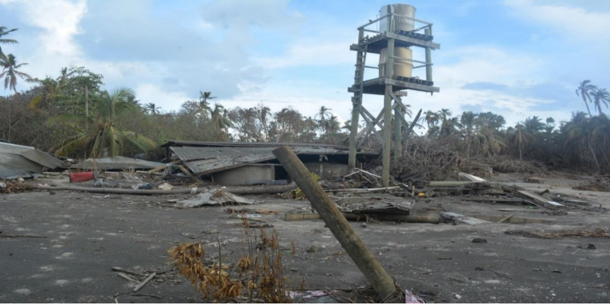
Pic: Damage from the tsunami on Fafaa Island. Source: MEI DECC
