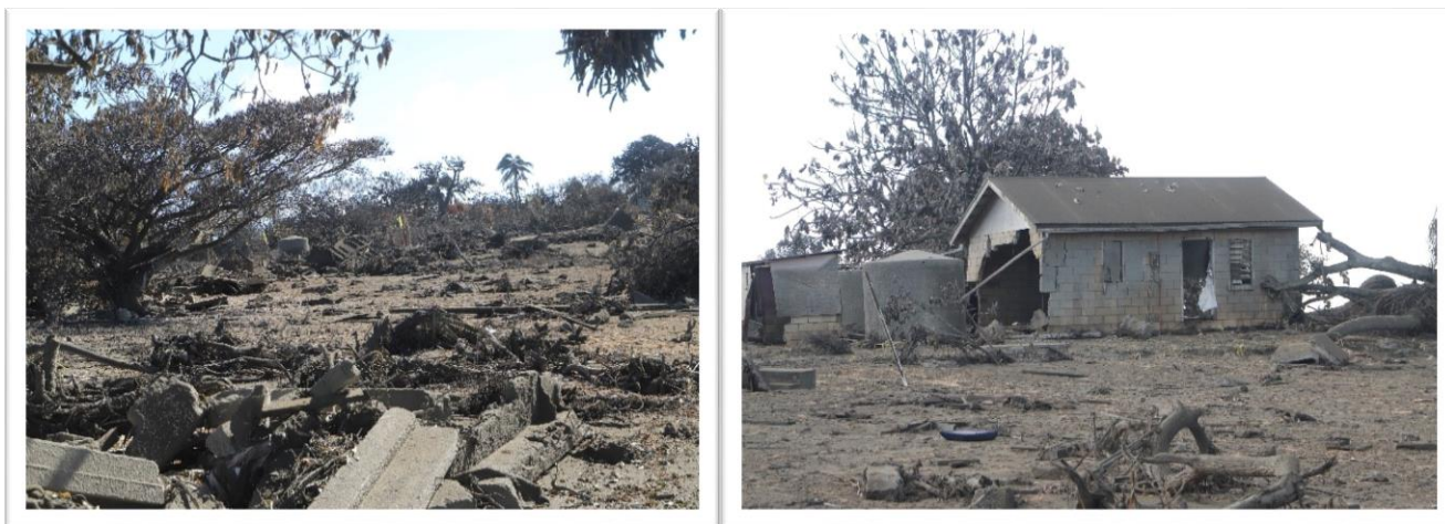
Pic: Damaged houses and properties in Ha'apai Islands (Source MEIDECC)
