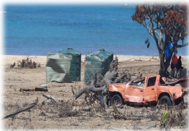
Pics: the fiber water tanks that has been damaged at Nomuka by the tsunami
